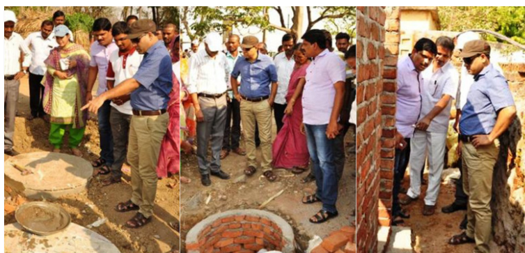
Toilet-construction campaign in Vizianagaram district | Source: The News Minute
